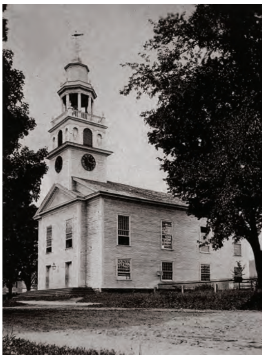
Old South Church prior to the 1922 alterations
